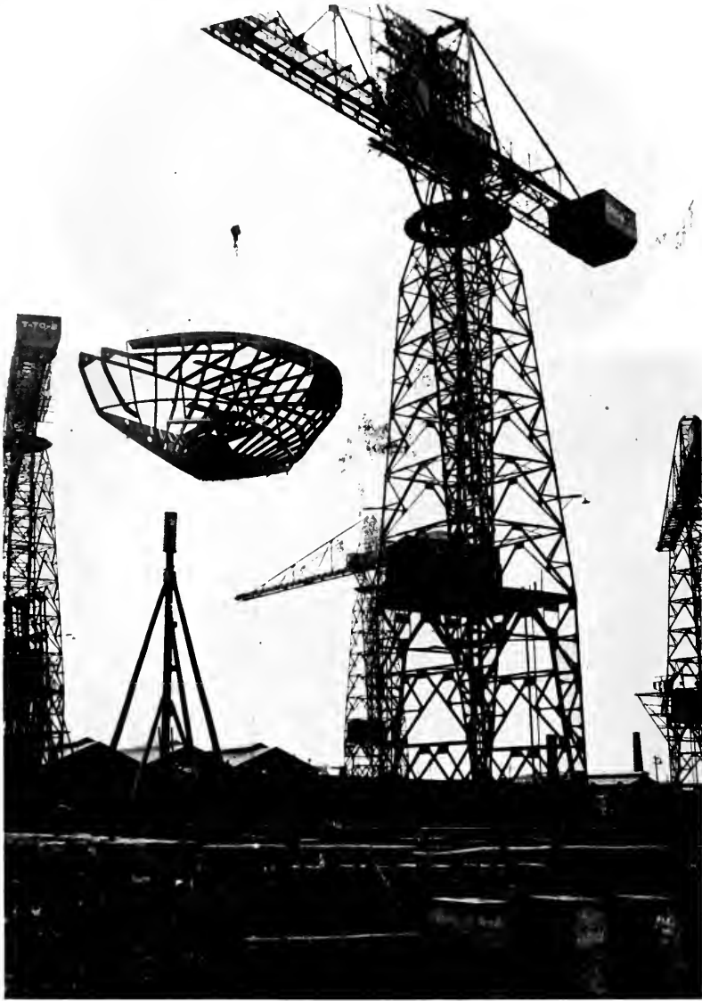
This picture gives an excellent idea of the extent and capacity of the crane equipment in this great Japanese shipyard. The crane in the foreground is handling the counter framing for a large steamer.
